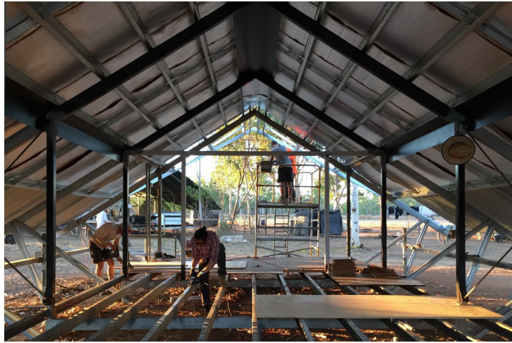
Figure 105: Ranger's accommodation under construction. The existing steel structure and foundations have been reused and incorporated into the new buildings. The roof has been updated with reflective insulation (AIR-CELL Insulbreak) and a ventilated cavity to provide better protection from the sun.
