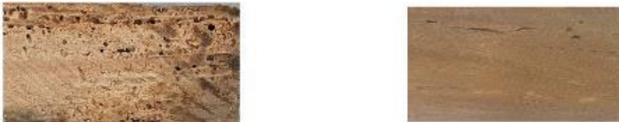
Figure 40: A) Section through timber post infestation. B) Mild timber infestation. (Source: Graham, 2022)
