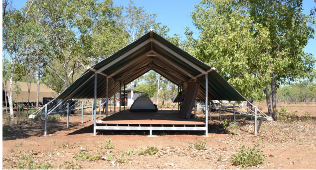
Figure 103: One of the original bala balas, consisting of a steel frame, raised timber deck floor and tarpaulin roof.
